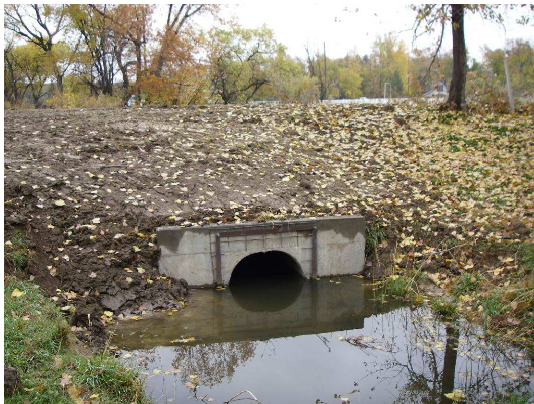
Figure 36. Conveyance for Leyden Creek Beneath the Croke Canal (After Repairs)
