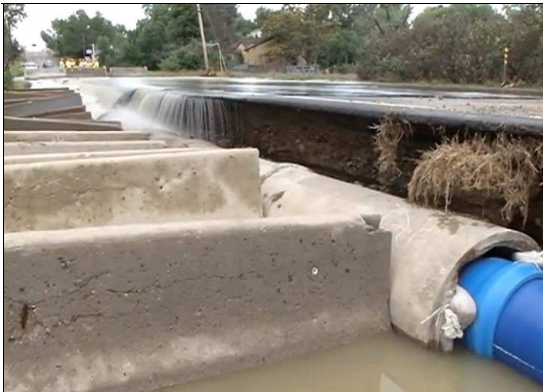
Figure 28. Water Main Damage at Indiana Street (Looking South East).
