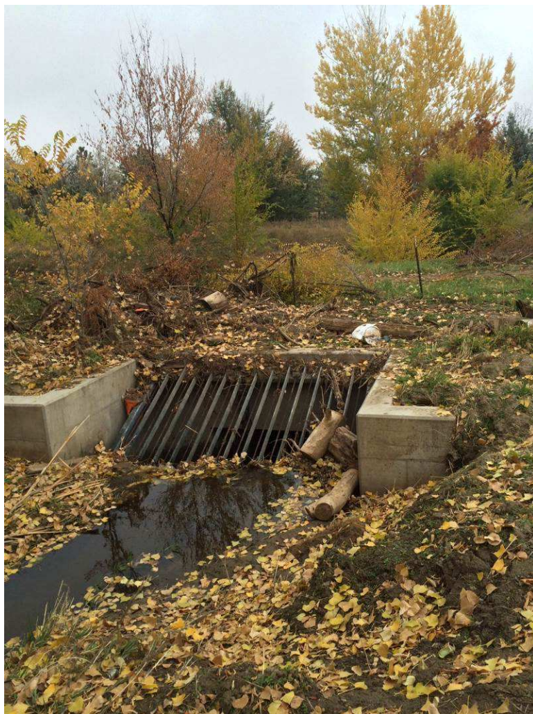
Figure 7. Entrance to Siphon Conveying Van Bibber Creek beneath the Croke Canal.
