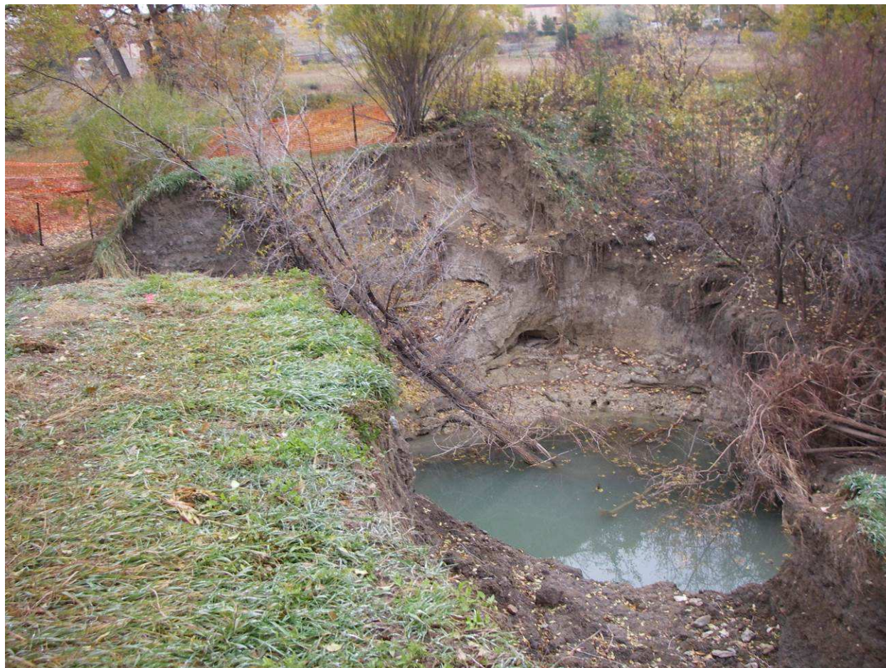
Figure 24. Leyden Creek Breach of the Church Ditch Upstream of Leyden Reservoir.
