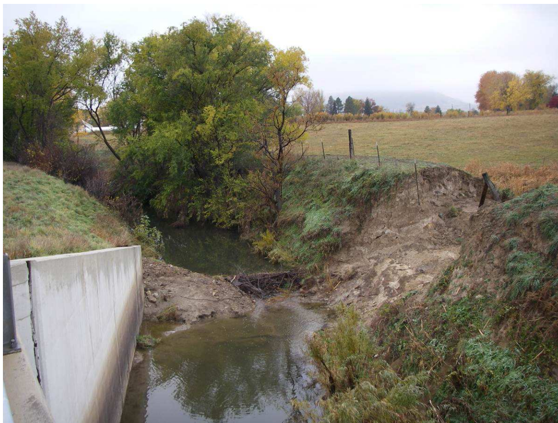
Figure 10. Moon Gulch Breach into Croke Canal.
